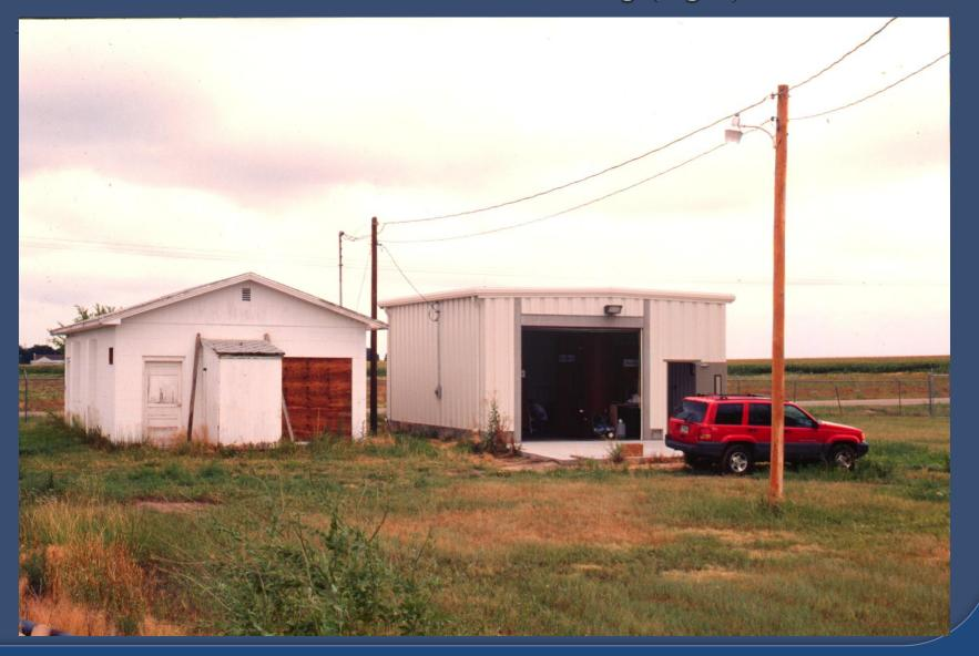
Wiggins demonstration plant: (right) anoxic denitrifying biotowers and aerobic prefilter; (left) slow sand filter.
