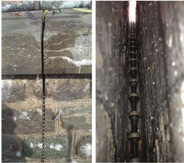
Figure 3.196: The slot cutting from downstream face. On the left, the kerb of the crest; on the right, the wire in the middle of the cutting; Sbarigia, Zinetti, and Hernandez-Bagaglia (2016)
