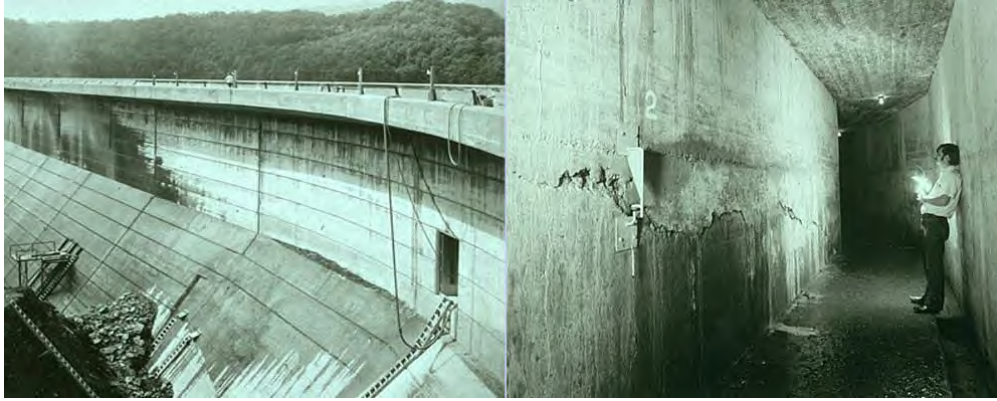
Figure 3.30: Fontana Dam, left abutment: views of the cracked surface (a discontinuity in water flow pattern can be noticed in the photo) and inside the inspection gallery (after Ingraffea (1990)); Comi, Fedele, and Perego (2009)
