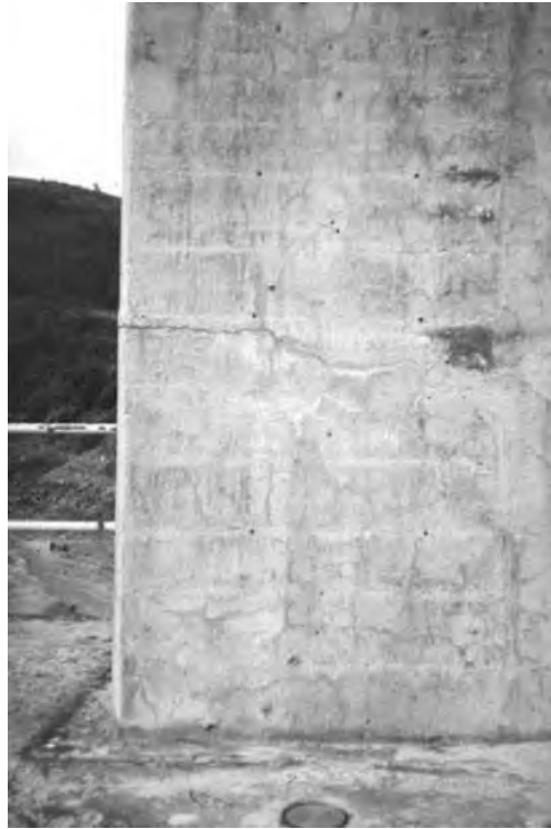
Figure 3.114: Map-like fissures on a concrete wall in the Belesar Dam; Herrador, Martínez-Abella, and Dopico (2008)
