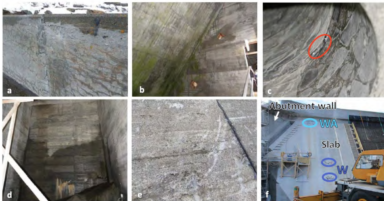
Figure 3.175: Photos of the Votna I Dam: a) map cracking at the rail of the Dam; b) map cracking inside the slab ; c) presence of ASR gel in a bore hole; d) humidity inside the slab; e) aggregates visible on the surface; f) upstream face after drilling; Plusquellec et al. (2018)
