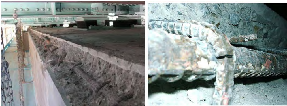
Figure 3.146: Chipping inspection of pier beam (left); Fractured steel bar (right); Miyagawa et al. (2006)
