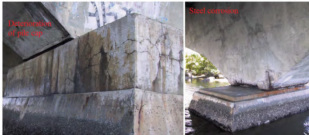
Figure 3.111: Signs of deterioration at the Paulo Guerra Bridge (left); severe steel corrosion (right); Helene, Carvalho, and Pacheco (2017)
