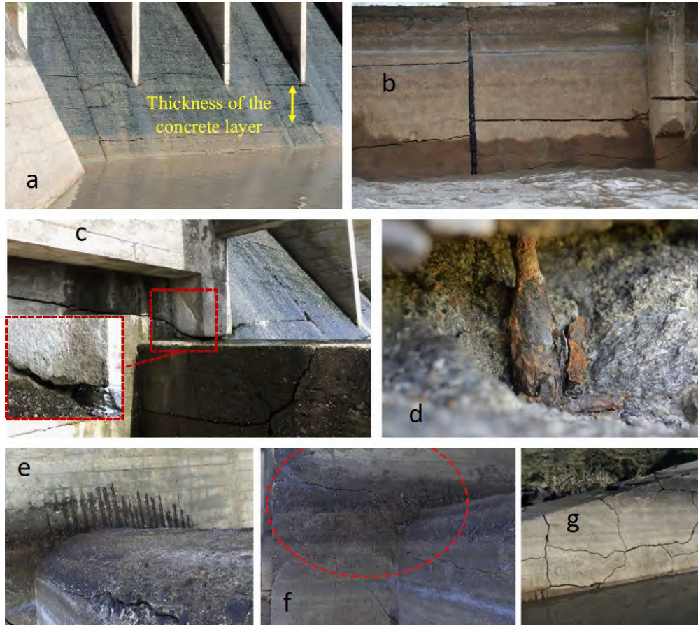
Figure 3.19: Observed damages: (a) cracks in downstream face, (b) crack of upstream face, (c) cracks of strainway and loos of concrete, (d) corrosion of rebars, (e) erosion in diaphragm, (f) cracks in diaphragms, and (g) map cracking in the retaining walls of the dike; Blanco et al. (2018)
