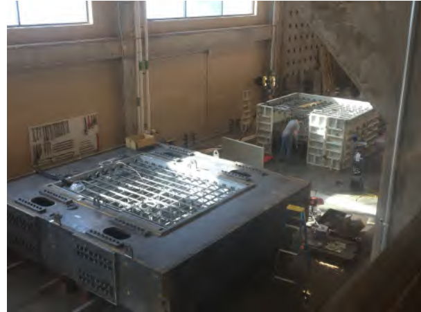
(b) Form construction
