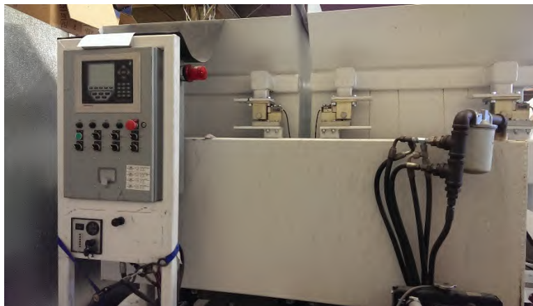
Figure 109 - Close view of mobile batch plant at Fall Line. Note load cells for weighing hopper contents.
