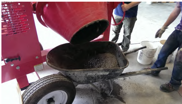
Figure 56 - Discharging freshly-mixed concrete
