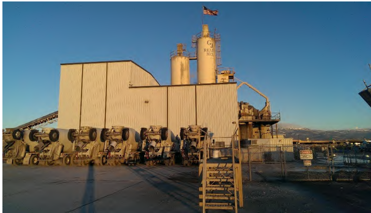
Figure 3 - Grand Junction Ready Mix, Grand Junction, Colorado
