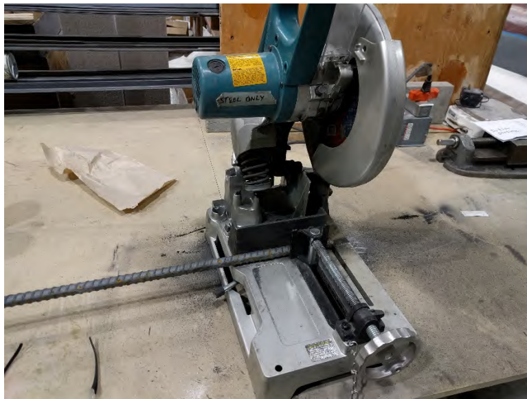
Figure 100 - Cutting reinforcing bar
