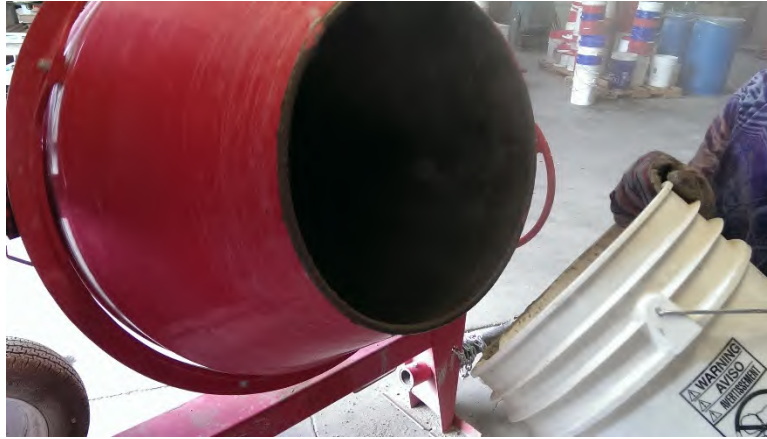
Figure 54 - Charging the mixer
