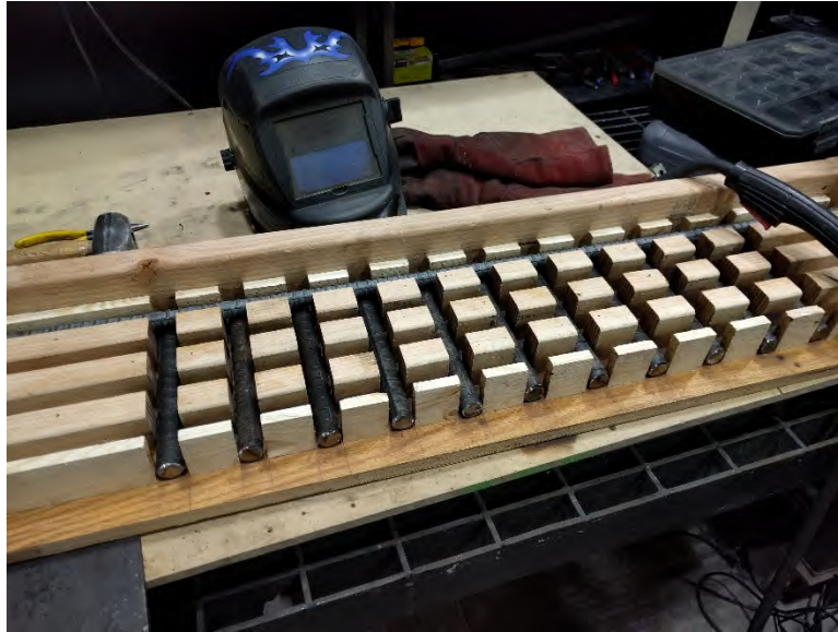
Figure 101 - Rebar layout and welding using the wooden jig.
