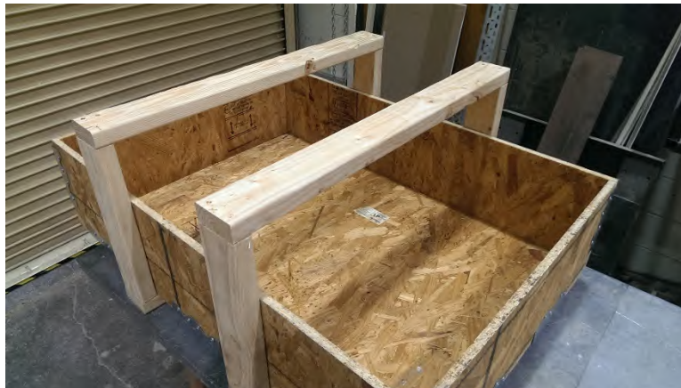
Figure 104 – Example shear specimen formwork
