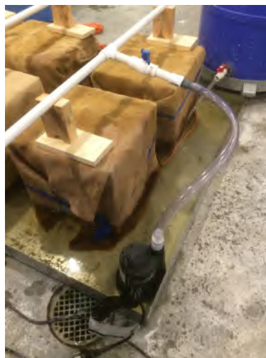
Figure 2.16: Sump pumps used to power sprinkler system
