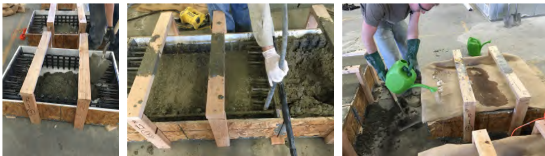
Figure 2.9: Filling forms, vibrating concrete, and covering with wetted burlap
