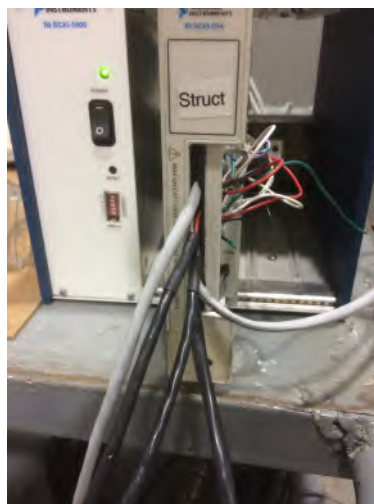
Figure 4.1: Connections from SCXI-1314 terminal block
