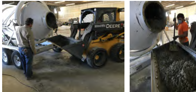
Figure 2.7: Pouring mixed cement from mixer for testing and transportation to forms
