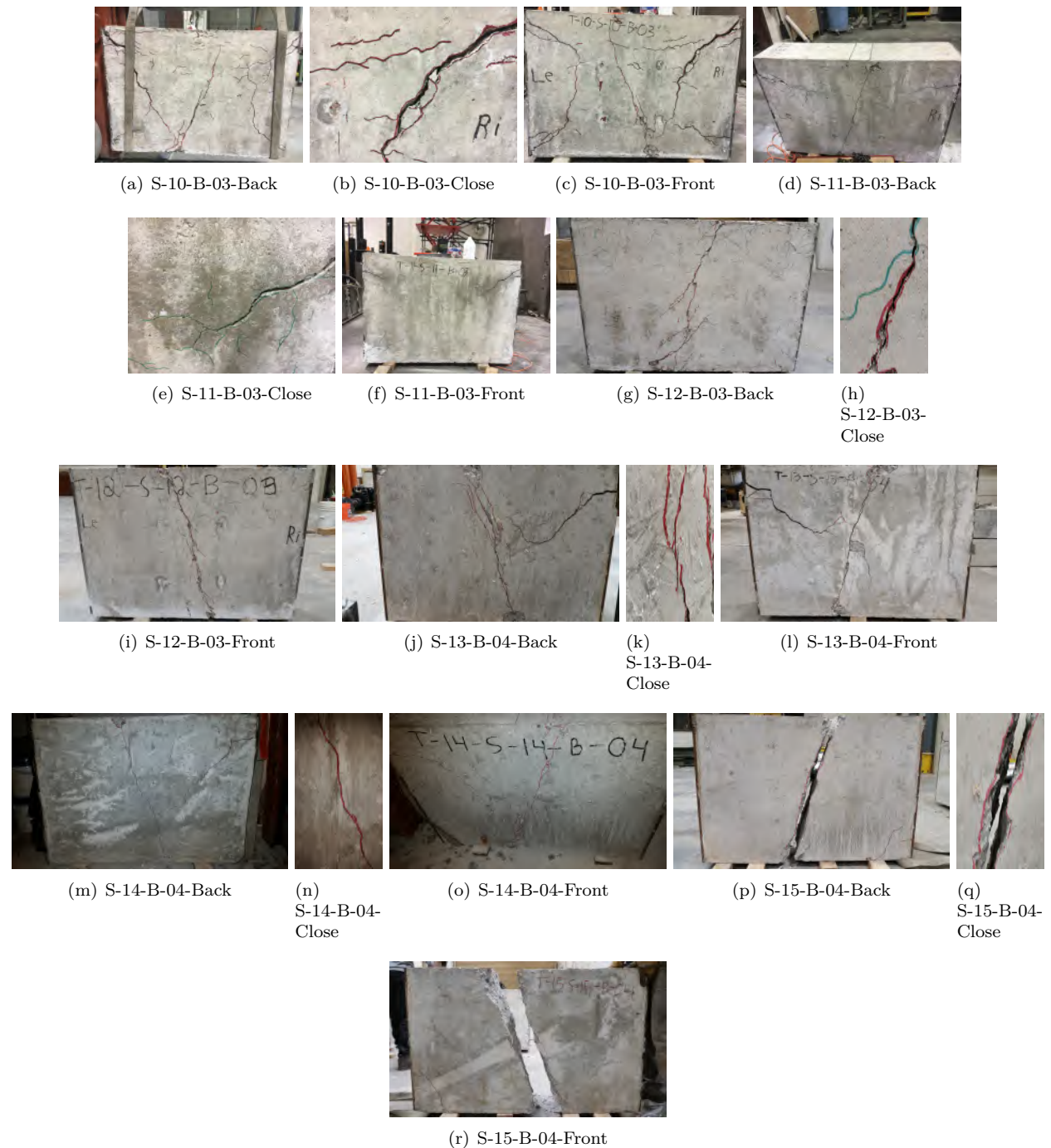
Figure 5.2: Post-Mortem pictures of specimens 10 to 16
