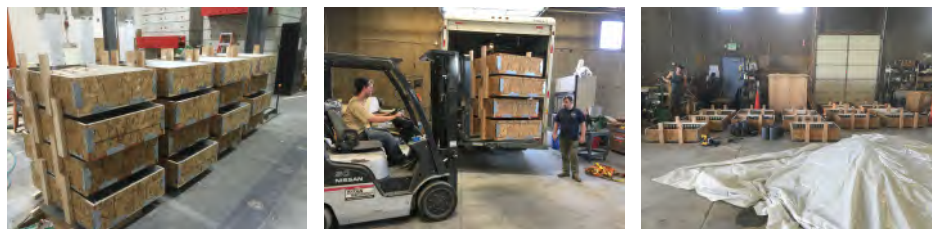
Figure 2.3: Wood forms built, transported, and organized at casting location
