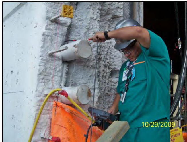
Figure 4: 5" tendon conduits (Progress Energy Florida (ML102861026), 2009)
